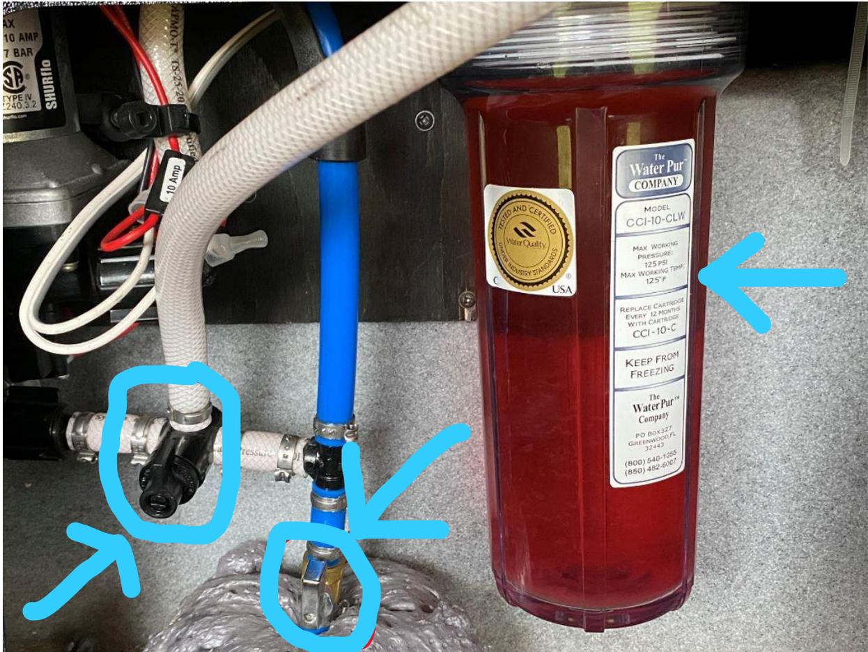
Below is an image of the hot water tank by-pass levers. This is located under the kitchen sink. To access these levers you must remove the second drawer (From the top).
